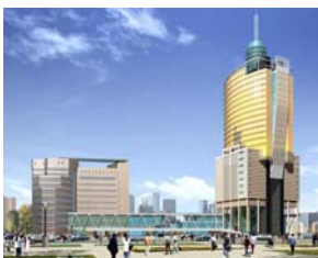
ZhuHai Telecommunication Building
