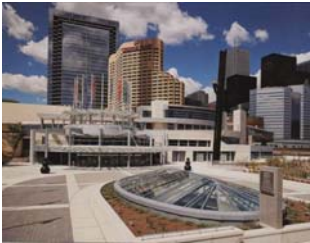
Metro Toronto Convention Centre Expansion
