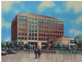
Regional Municipality of Waterloo Building
