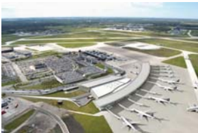
Winnipeg James Armstrong Richardson International Airport
